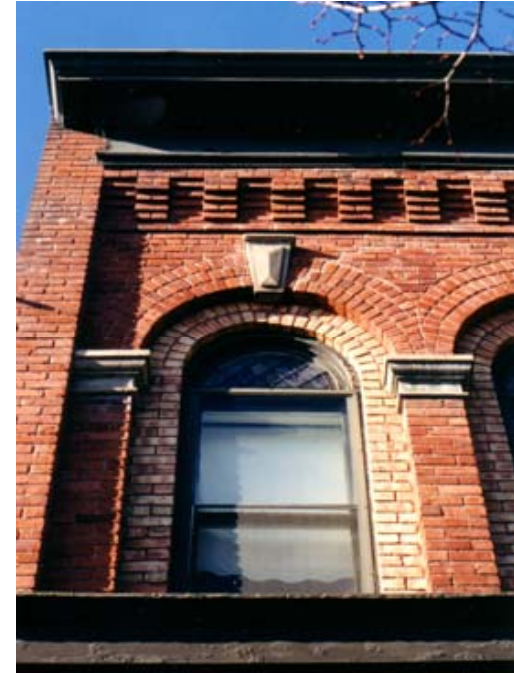
The cornice forms a definitive element at the top of the façade. It may be very deep, as above, or a relatively shallow construction, with pattern as its prominent characteristic. Both examples are from Collingwood.
