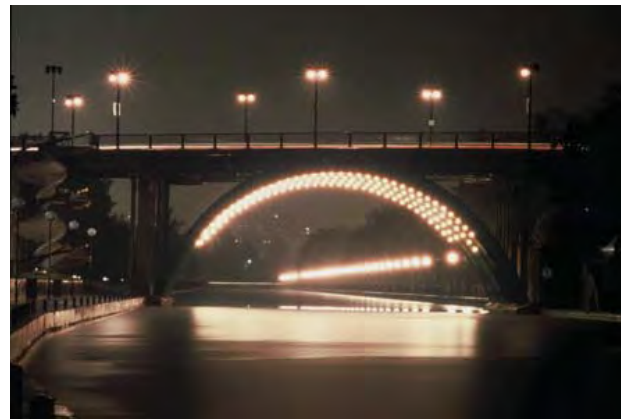
Rideau Canal: Low intensity globes on pedestrian scale lights outline the canal as they give excellent light to the pathway. Low pole acorn lights define the road with minimal illumination. Silhouette reveals soft landscape and highlights make the bridges stand out as orientation points.
