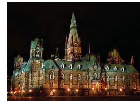
After implementation of the lighting strategy, the West Block softly glows as a background feature. This allowed good visibility and resulted in a clear emphasis on the entrance and architecture. Light is provided at the entrance, on the lower façade from pedestrian scale lights and above from lights hidden on adjacent rooftops.
