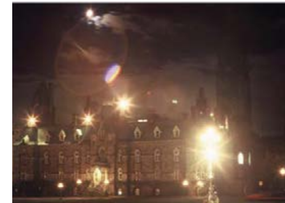
West Block, Parliament Hill: Glare vs. Visibility - Before lighting improvements, roof mounted security lights caused glare that was so bright in contrast to their surroundings that vision was obscured, blocking the view of the building and making it generally more difficult to see.
