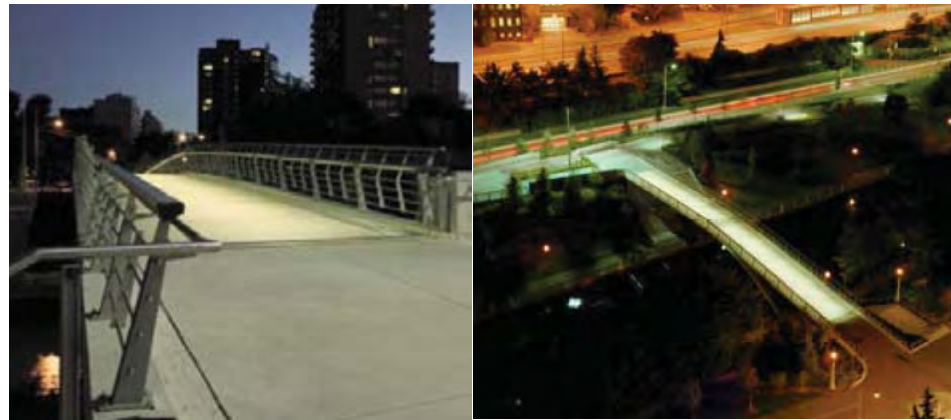
Cork Town Pedestrian Bridge: Soft light floods the bridge floor from glare free LED lighting in the handrail, allowing comfortable recognition of surfaces and spectacular views down the Rideau Canal.
