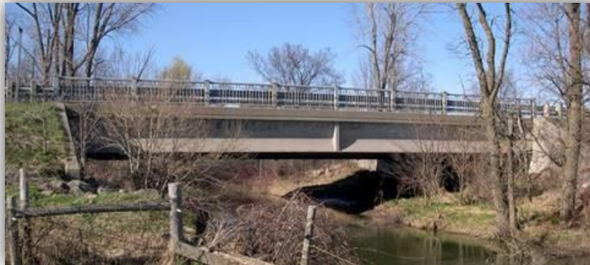
Figure 38: Girder Bridge Illustration
