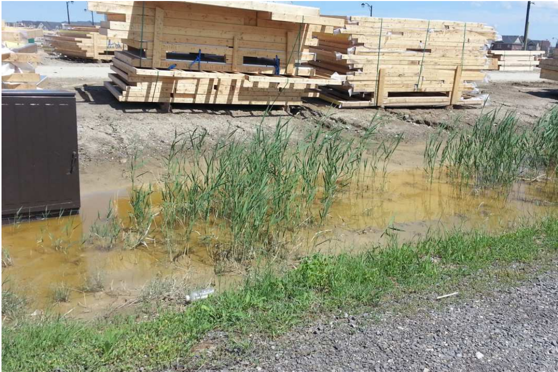
Photo 10: Standing water at the ditch of the road
