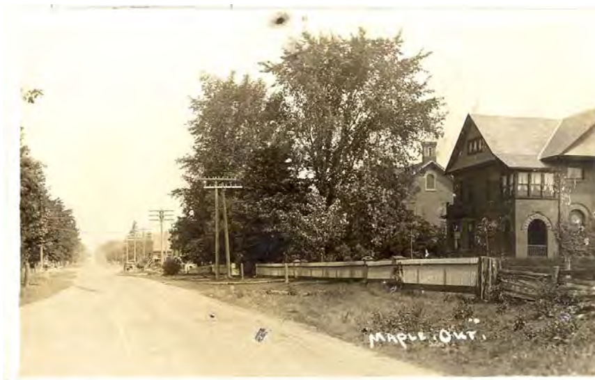
A very substantial picket fence is seen in front of the James Kirby House at 9983 Keele Street. Photo from the Vaughan Archives
