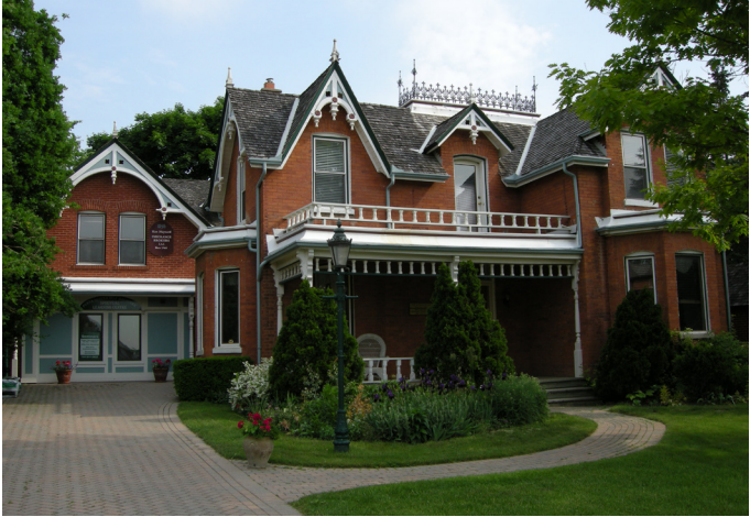
Heritage Building - Woodbridge Avenue
