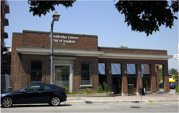
Heritage Building - Woodbridge Avenue
