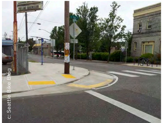
Figure 4.60. Mountable truck apron.
