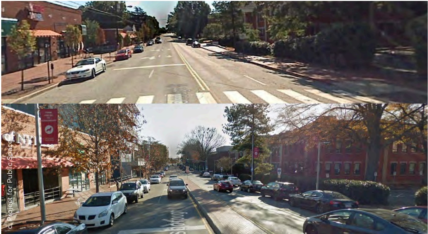
Figure 4.19. Rightsizing Hillsborough Street (City of Raleigh, NC) resulted in a 23% decrease in vehicle crashes. It involved reducing four travel lanes to two, adding on-street parking, cycle lanes and a median, and widening sidewalks.
