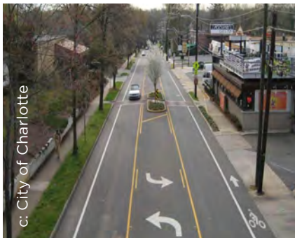
Figure 4.17. Lane reduction and conversion, addition of cycle lanes, medians and pedestrian refuge islands.
