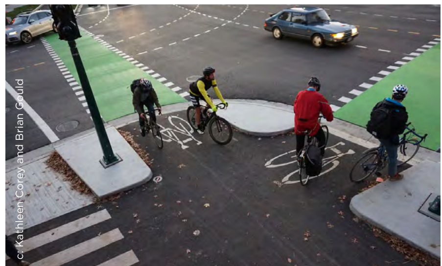
Figure 2.21. Protected intersections increase driver visibility of people in the crossride and crosswalk by setting back the crossride from the motor vehicle travel lane.
