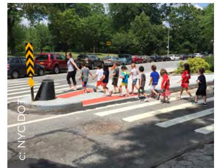
Figure 2.18. Median crossing reduces the crossing length and exposure to vehicle traffic for pedestrians.
