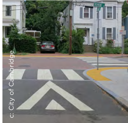
Figure 4.32. Raised crosswalk at intersection.
