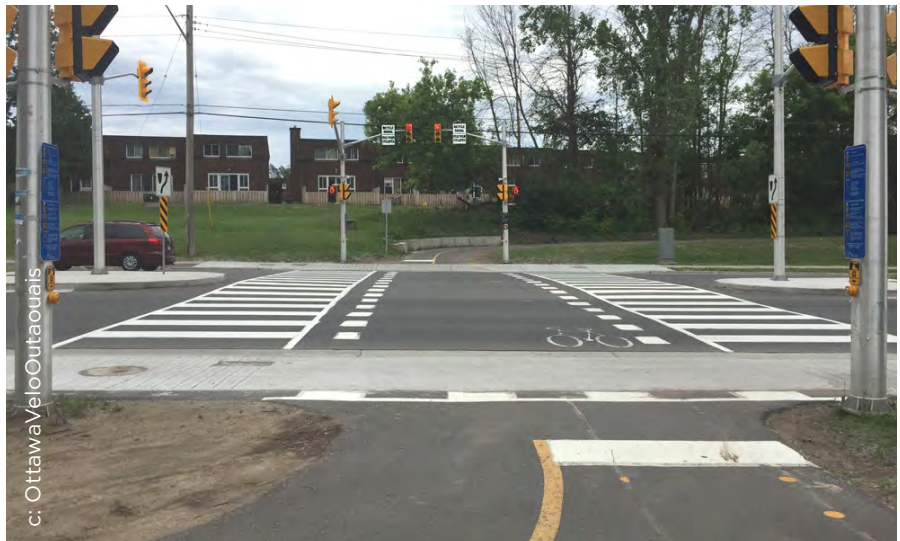
Figure 4.75. Midblock crossroad and bike signal for trail access.
