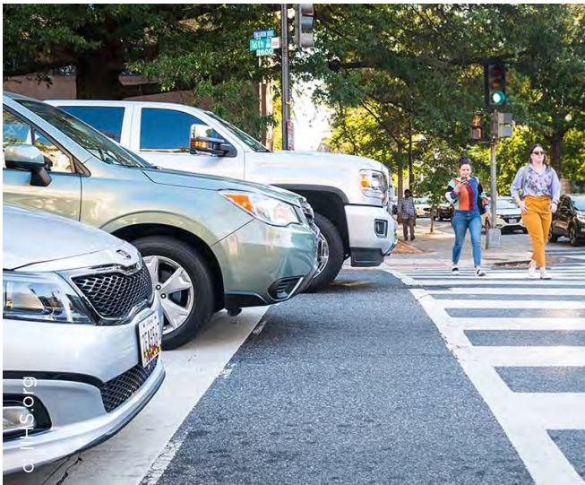
Figure 4.83. Large design vehicles encroaching on space between stop line and crosswalk.
