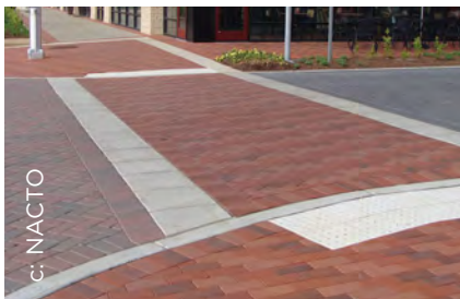
Figure 4.63. Raised driveway and the continuation of the paving material over the driveway highlights crossing of different users.
