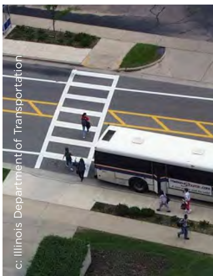
Figure 2.20. Midblock crosswalks facilitate crossing along desire lines across streets to transit stops, parks or schools.
