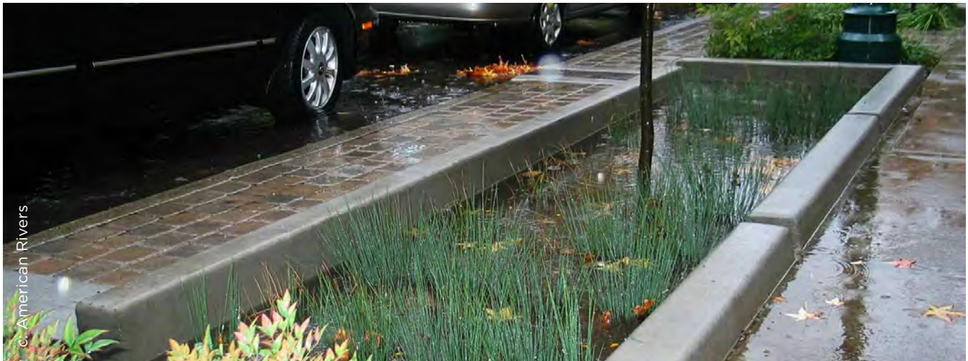
Figure 4.38. Stormwater management system: bioswale.
