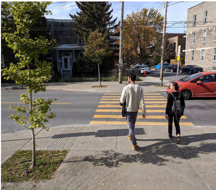
Figure 2.17. Curb extensions increase the overall visibility of pedestrians by reducing the crossing distance for pedestrians.
