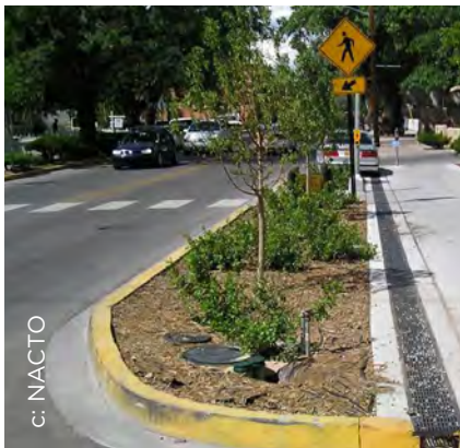
Figure 4.34. Midblock curb extension.
