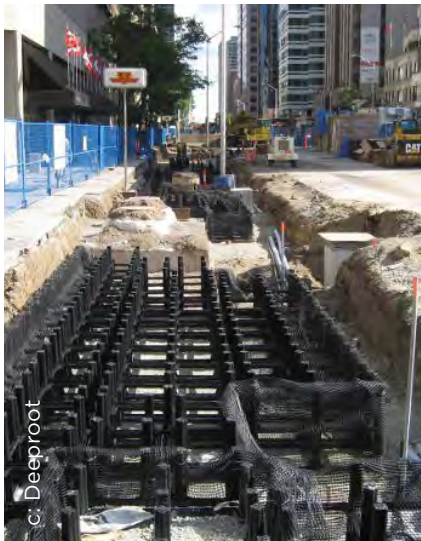
Figure 4.45. Soil cells (Bloor Street, Toronto).
