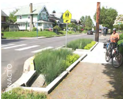
Figure 4.42. Permeable paving with rain garden in curb extension.
