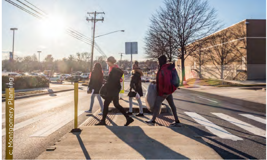
Figure 4.68. Pedestrian refuge with vertical elements and signage.
