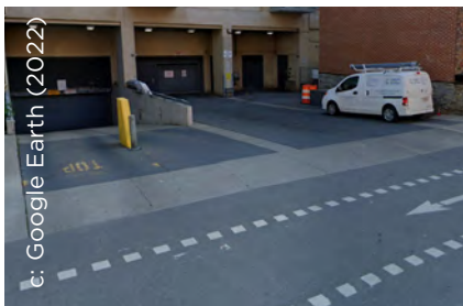
Figure 4.62. Raised driveway into parking garage.
