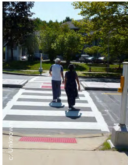
Figure 2.27. Midblock crosswalks facilitate crossing along desire lines across streets to recreational trails, transit stops and schools.
