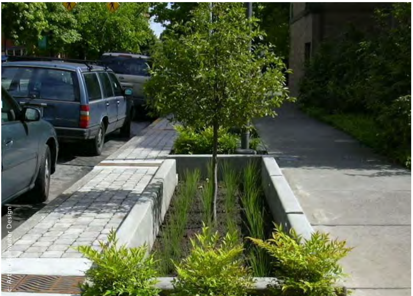
Figure 2.34. Different street tree planting details are available to ensure healthy growth: the most common are the soil trench (top left), soil cells (top right) and open planters (bottom). Further, each can provide stormwater management opportunities.
