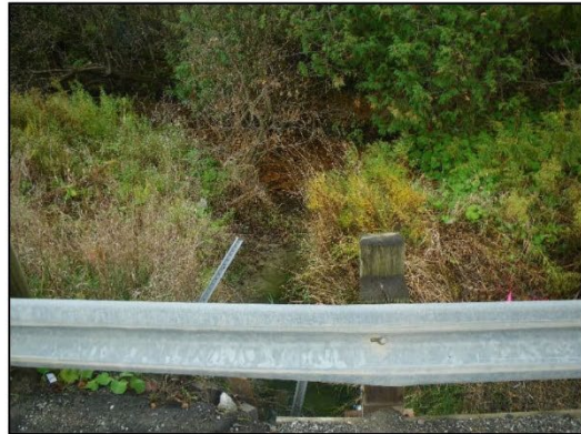
Downstream end of culvert facing downstream (south)
