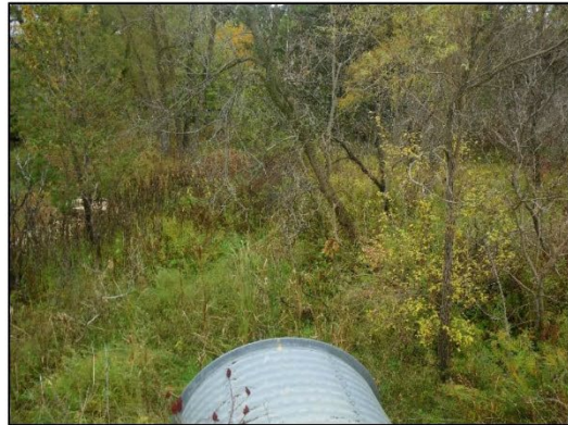
Downstream end of culvert facing downstream (south)
