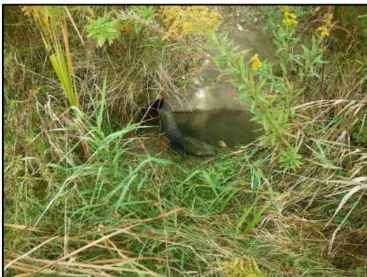
Downstream end of culvert facing upstream (north)
