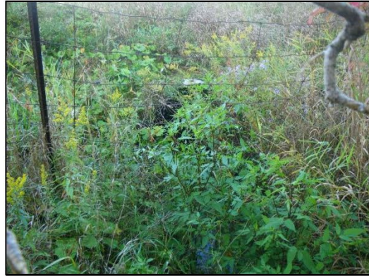
Downstream end of culvert facing upstream (north)
