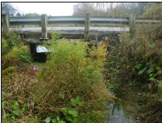
Downstream end of culvert facing upstream (north)
