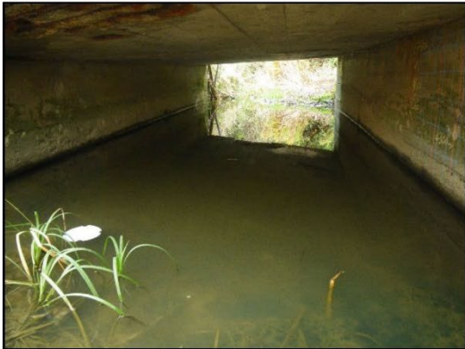
Pool through culvert at Crossing C2 facing downstream (south)
