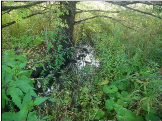
Defined channel downstream of culvert facing downstream (southwest)
