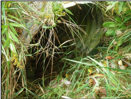
Upstream end of culvert
