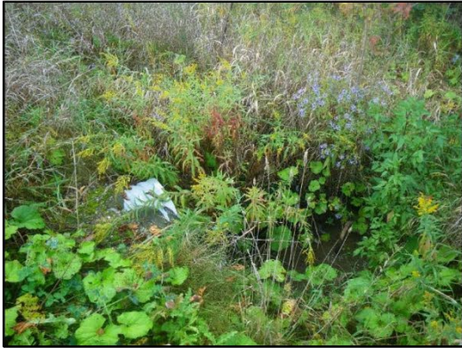
Downstream end of CSPA culvert facing east
