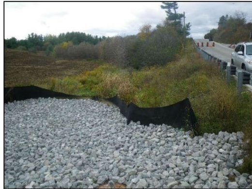
Swale downstream of culvert (outlet adjacent to cattails in center of photo). Note rip rap associated with a future storm water facility outlet. Facing downstream (west)
