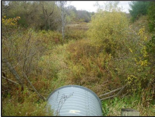
Facing upstream (north) from upstream end of Teston Road culvert
