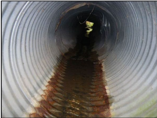
Facing downstream from upstream end of culvert under Teston Road.
