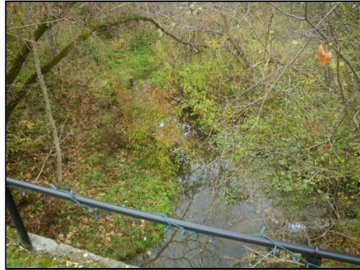
Channel downstream of Crossing C2 just upstream of where it abuts Teston Road slope at 5011 Teston Road. Photo taken from driveway facing upstream (southwest)
