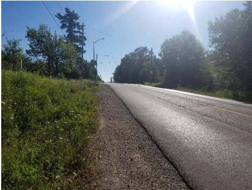
Plate 1: View of the study area with the narrow shoulder, looking east-northeast from west of Teston Road and Kipling Avenue.
