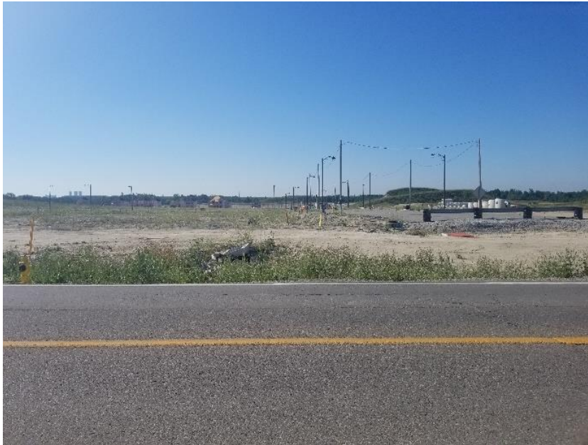
Plate 5: Large residential subdivision under construction south of the study area, looking south.
