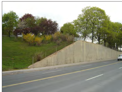
Concrete retaining wall east of railway bridge
