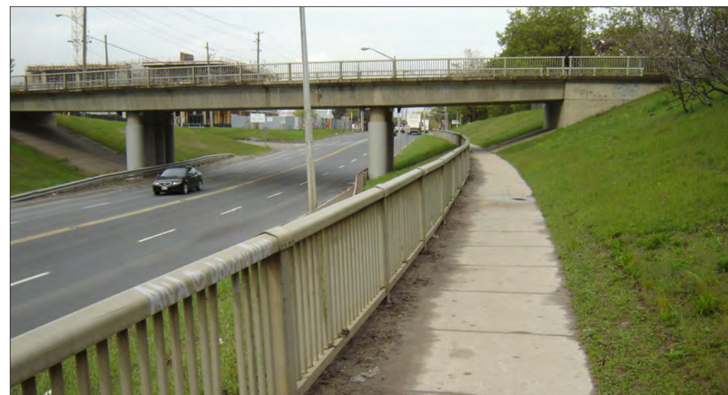
The railway bridge (looking west)
