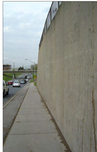
Concrete retaining wall east of railway bridge
