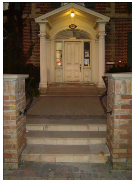
Existing entrance to Beaver Brook house
