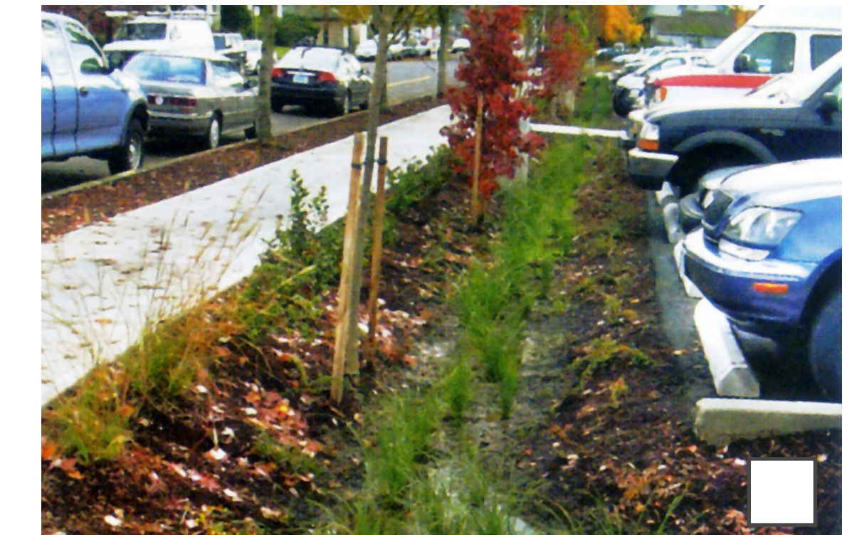
Bio-swales for on-site storm water retention.
