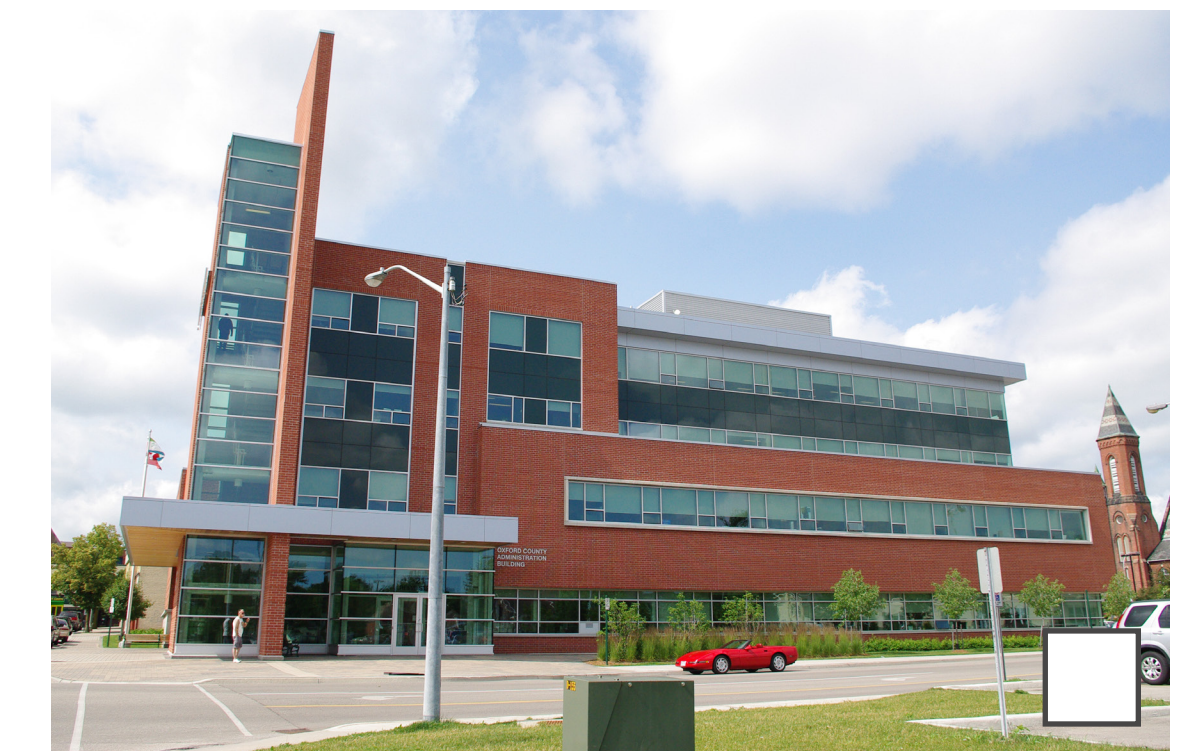
Government service buildings.
