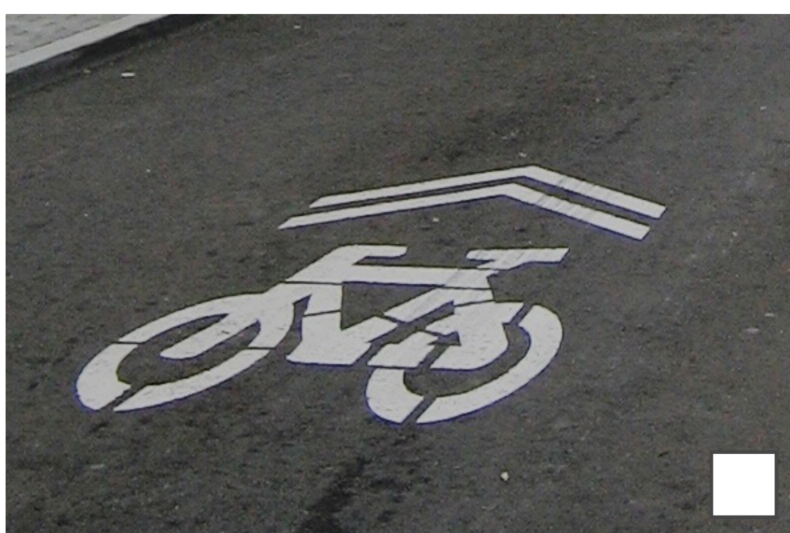
Streets with sharrow markings to accommodate shared vehicular and cyclist movement.
