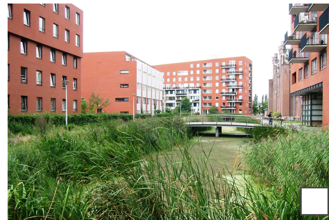
On-site storm water management and filtration.
