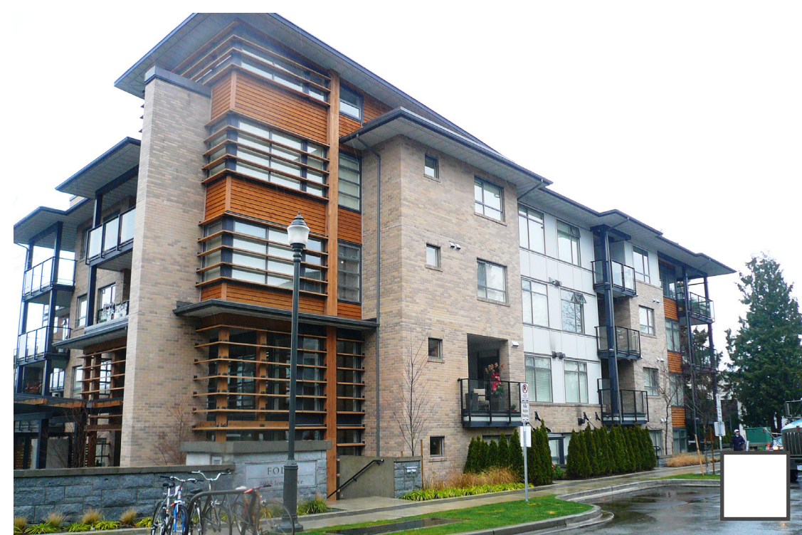
Low-rise residential apartment buildings and/or mixed-use buildings.
