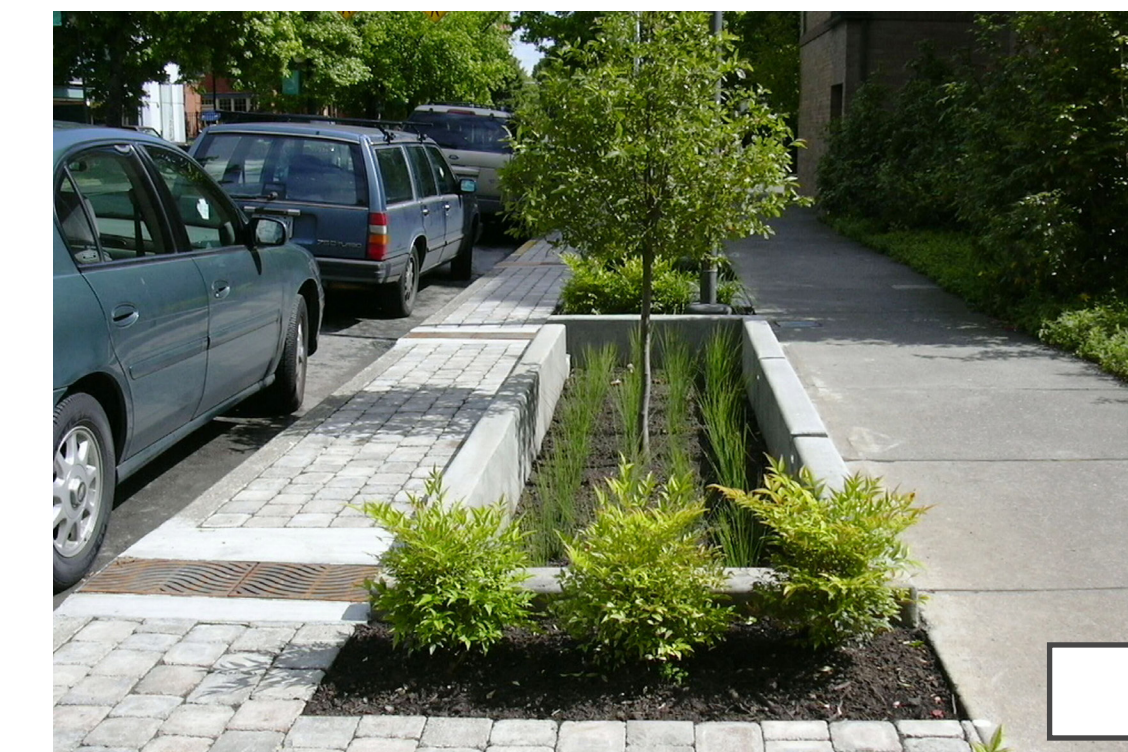
Boulevards designed for stormwater retention.
