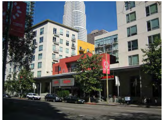
Figure 145. Retail hides truck docks and parking access on the back, Washington (Image Credits: Joe Urban)
