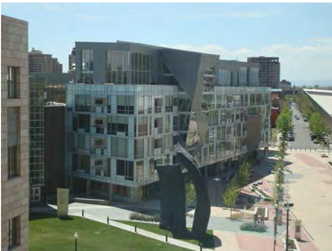
Figure 144. Multi-level parking garage wrapped with residential, Denver Art Museum Residences, US (image credits Henry Pesciotta)
