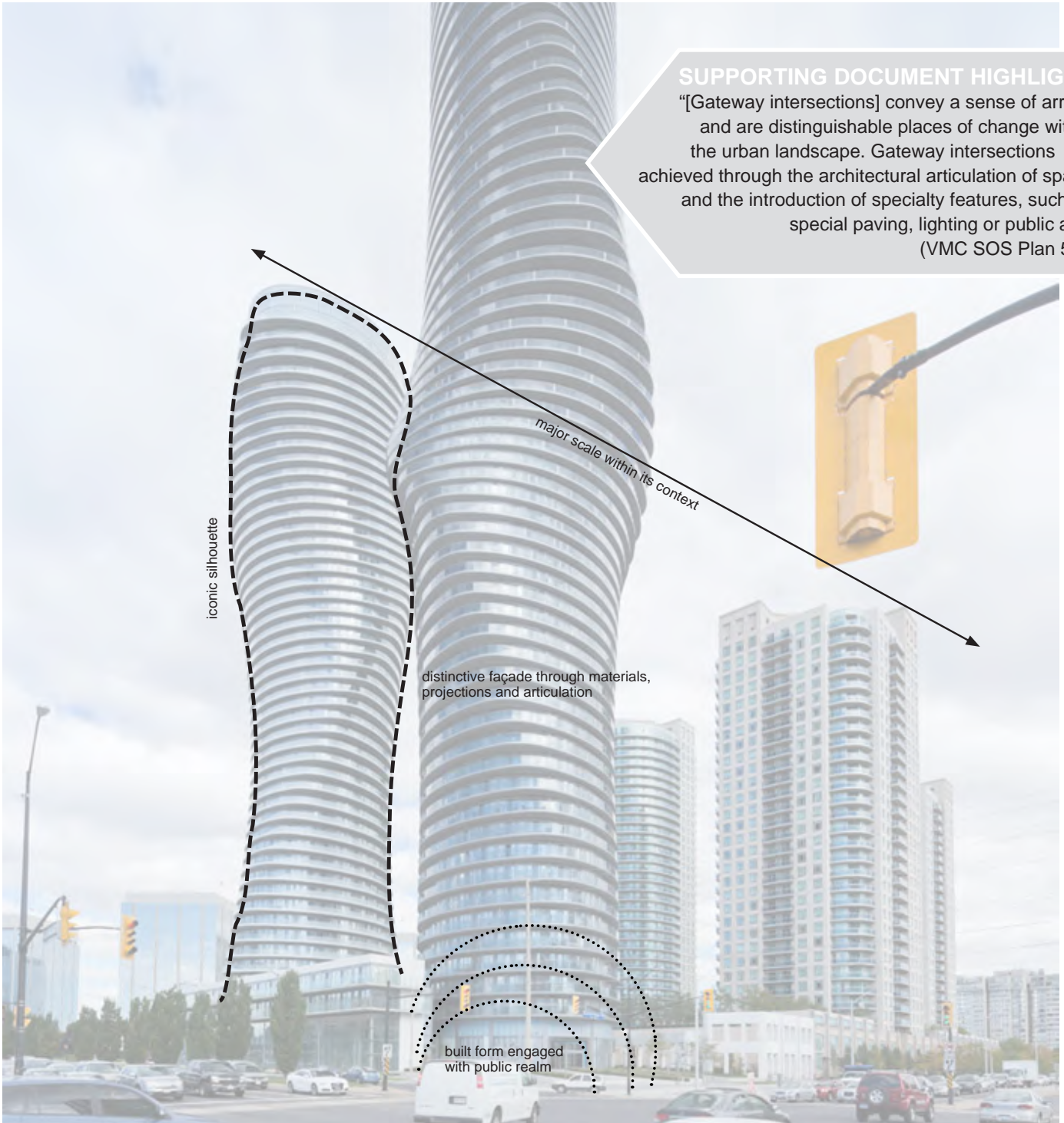
Figure 179. The Absolute Towers, Mississauga (Image Credits: Iwaan Ban)
