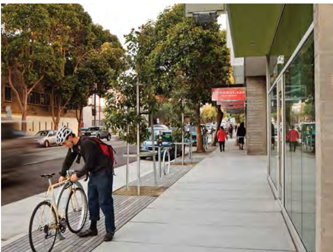
Figure 130. Gough street, permeable pavement, San Francisco (Image Credits: Bruce Damonte)
