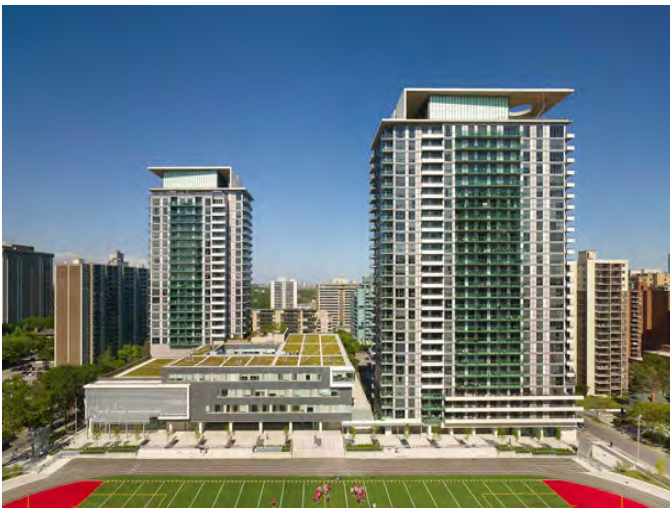
Figure 112. The Republic Condominiums, Toronto (Image Credits: Burka Architects)
