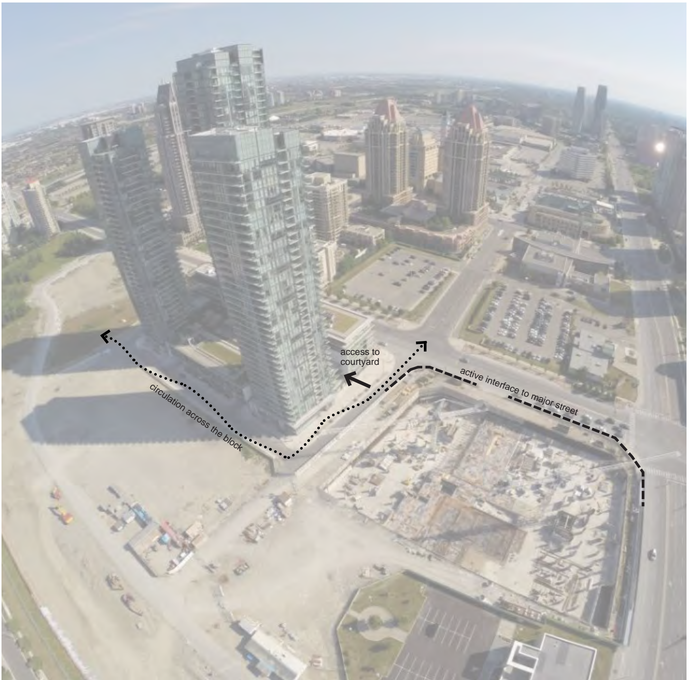
Figure 220. Aerial view of Parkside Village Residences (Image credits Jasonzed)
